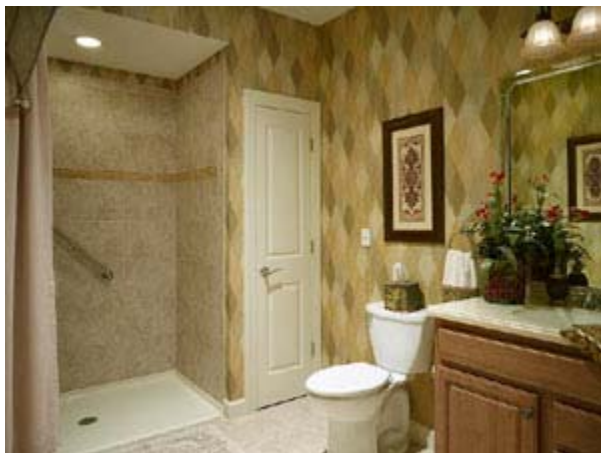
Grab bars are critical elements to sustained mobility and should be part of the planning process, as seen in bathroom at Fleet Landing's Villa model at the Palms.
